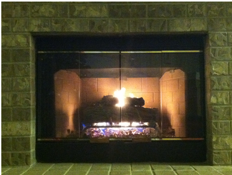
Figure 1 - A ventless combustion fireplace has no chimney; it draws combustion air from and releases combustion byproducts to the room in which it is located.
