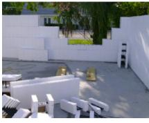
Interlocking pieces are used to create the ICF wall. Concrete is poured onsite into walls of polystyrene foam. Varying thicknesses and materials typically result in R-values between R-20 and R-45. Many times furring strips are used to allow cladding to be easily attached to the exterior.
