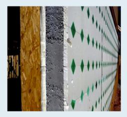
An ICF envelope can be finished with stucco, brick or other materials to produce a desired appearance and add to the aesthetic appeal, as shown below. However, due to the increased wall thickness, the building's footprint is greater than with some other types of framing.
