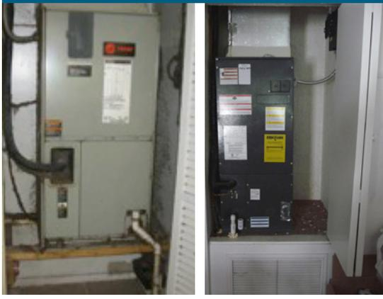
*(left)* The existing air handler was extremely leaky and mounted on a stand in the air handler closet. The closet was separated from the conditioned space by louvered doors, which restricted return air flow.
