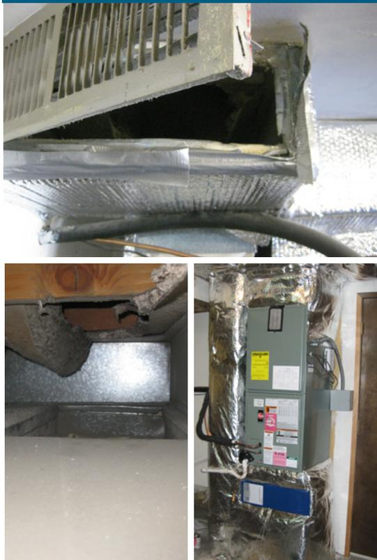
(top) Not only can faulty or poorly placed air returns (such as this one in the garage) allow air infiltration, they can also expose occupants to harmful pollutants.
